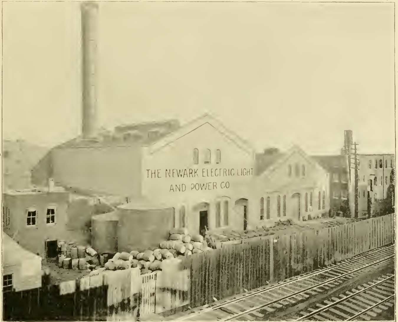
THE ELECTRIC LIGHTING PLANT ON THE PASSAIC RIVER.
